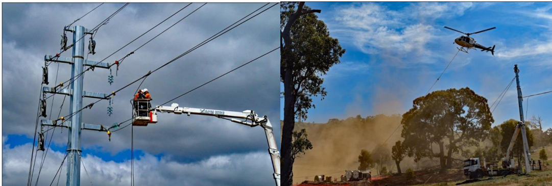
Stringing powerlines with the assistance of a helicopter
