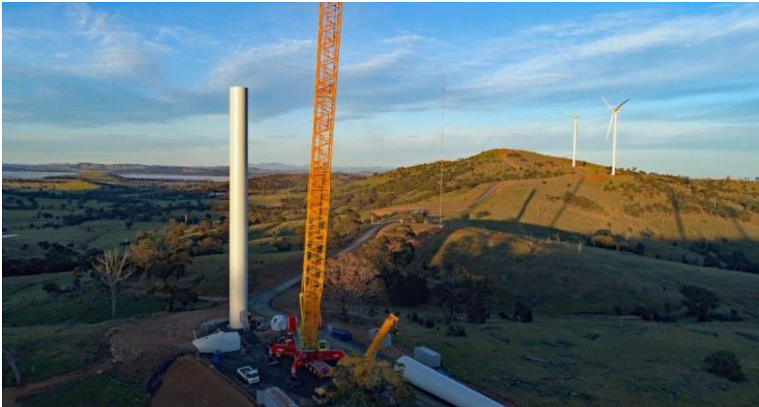
Sunrise over the site, showing towers being assembled
