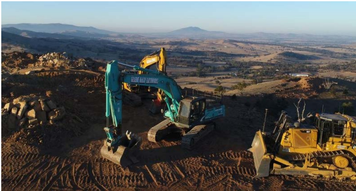
Sunrise over the site, showing civil works
