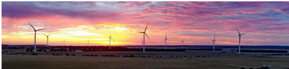
Sunrise over the completed project.
