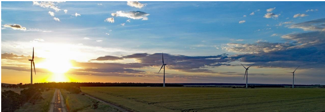
Sunrise over Glenmore Road, with turbines 5, 6, 7, and 8 assembled.
