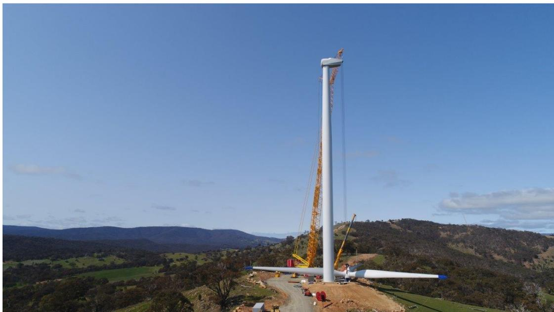
**The first turbine nears completion with blades and hub (the rotor) being assembled.**
