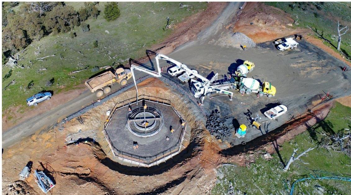
**Concrete foundation being poured.**
